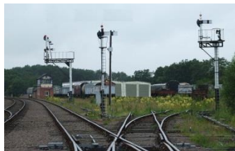
Shed location to the rear of existing sidings
